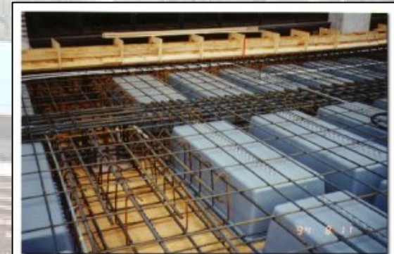
Example: Wide Module Concrete Joist Floor System
